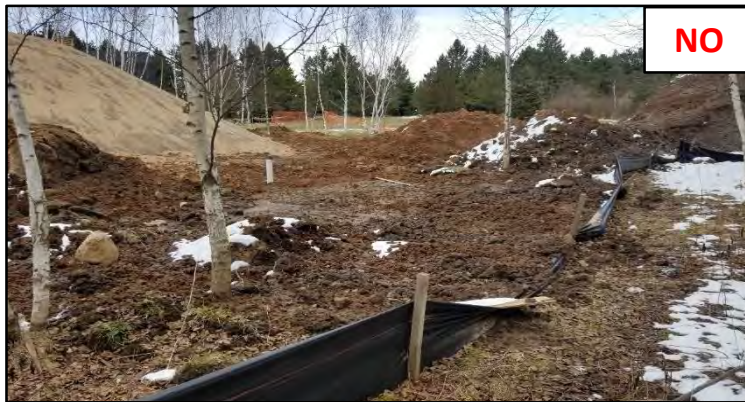
Fence sagging, run over by equipment.
