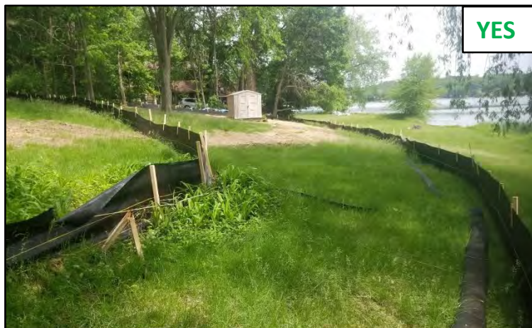
Double layer of silt fence with grass buffer next to Big Marine Lake.
