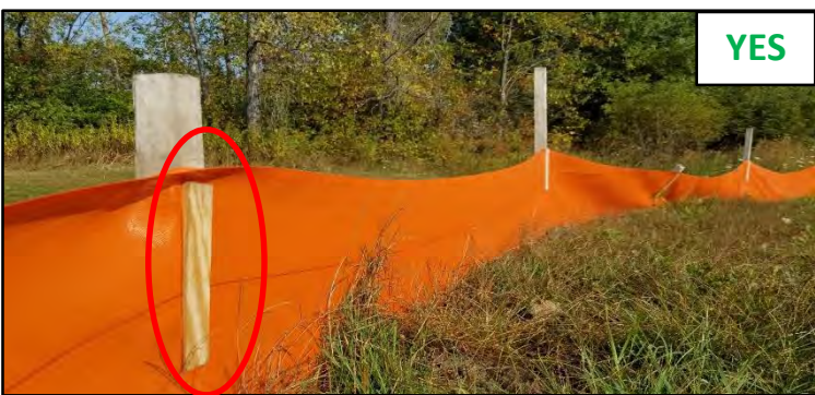
Fence tight, trenched in , secondary piece of lathe used for reinforcement.
